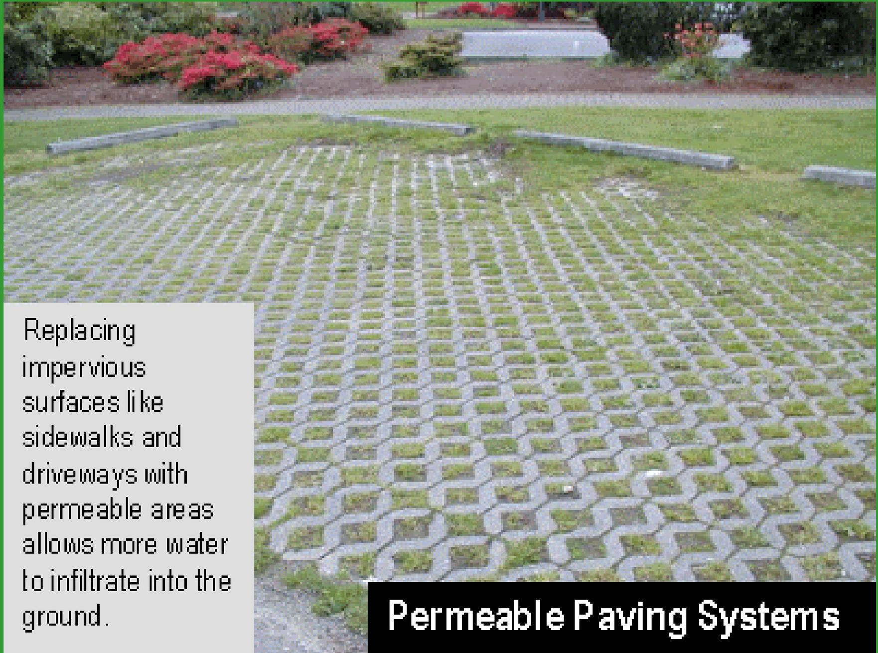
Replacing impervious surfaces like sidewalks and driveways with permeable areas allows more water to infiltrate into the ground.
